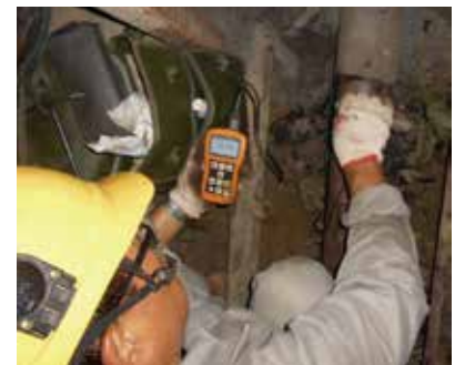
Soil and pipeline thickness analysis
